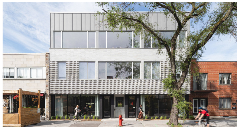
The front façade features St-Marc limestone that's used both in split-face format, placed at a 45 degree angle, as well as regular brickwork.
